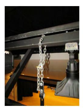
7.1.4. The support chains attach to plugging strip hangers without the top pipe This condition can stretch or elongate the hanger under load. A pipe should be inserted into these hangers.
