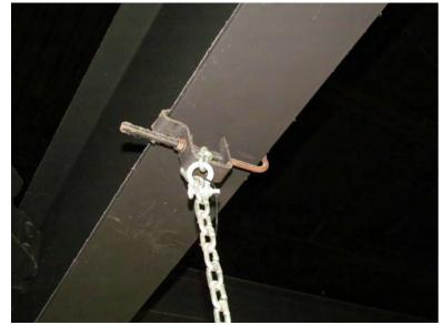
6.2. A number of the support chains are wrapped incorrectly around the battens, creating a crushing force on the chains. The chains should be wrapped around the battens without crossing over top of themselves.
