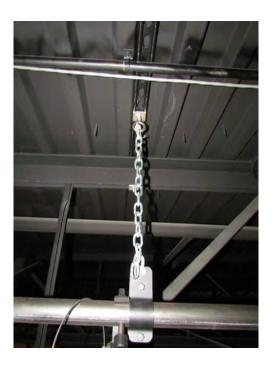
7.1.3. The ends of several trim chains are captured incorrectly in the termination rapid link. The dead-end links of the trim chain should be below the link.
