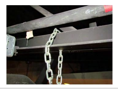
7.1.2. Unistrut® nuts are used to attach the shouldered eyebolts to the Unistrut® members. Unistrut® nuts are not recommended as there is no ensuring the nuts stay tight.
