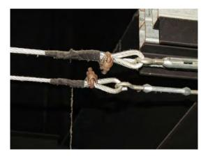
5.1.2. The wire guides are tensioned using light duty turnbuckles with unclosed eyes and hook ends. These turnbuckles should be replaced with jaw-to-eye turnbuckles with a known load rating.
